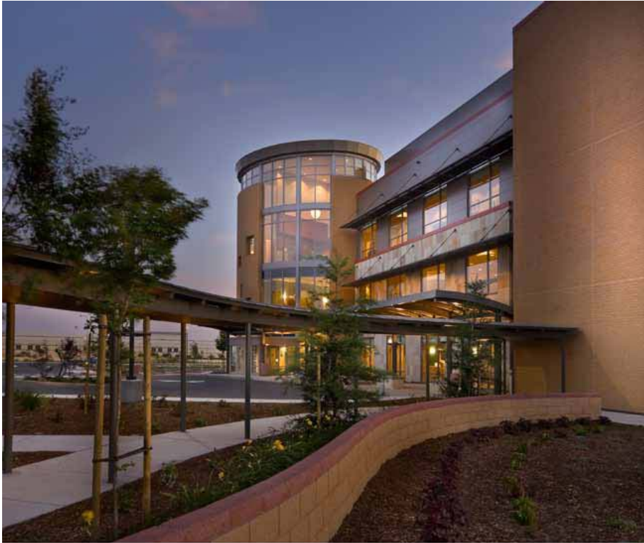
Figure 2: IPD project at Sutter Health Fairfield Medical Office Building (© Vance Fox)
