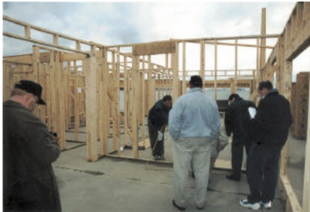
Figure 1 An example of a physical mock-up (PMU) used for a design review session (courtesy of Pulte Homes, Inc.)
