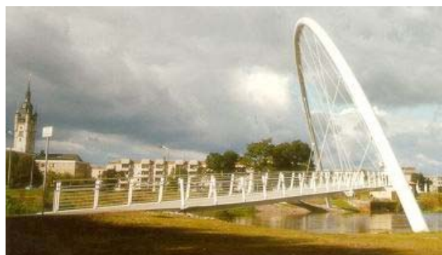
Figure 2 Arched bridge over the river Mulde in the city of Dessau (Germany)
