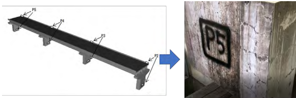
Fig. 5: Spray marking example, assuming the bridge piers inspection.
